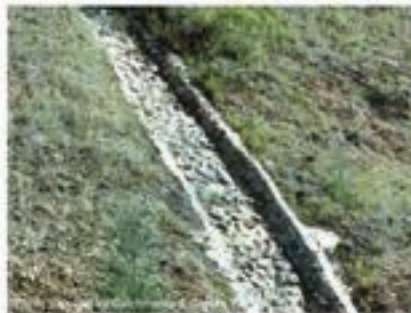
Photo 1 – Permanent, grouted-stone batter chute
