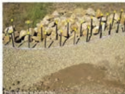
Photo 6 – Upstream face of a sediment weir
