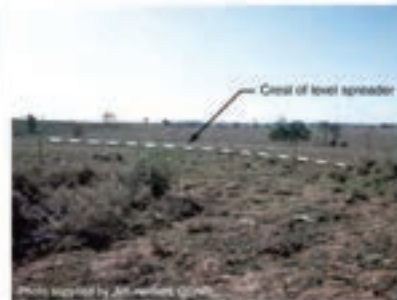
Photo 2 – Level spreader established to discharge stormwater from a diversion drain into the roadside property
