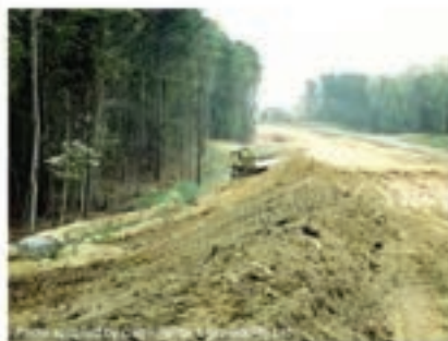
Photo 1 – Tracked vehicle walking up and down slope
