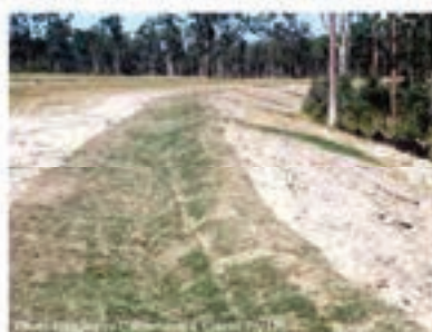
Photo 6 – Turf-lined flow diversion bank with grass-lined outlet chutes at regular intervals along the embankment
