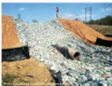
Photo 1 – Rock-lined sediment basin spillway with low-flow pipe outlet
