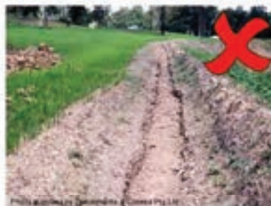
Photo 6 – Velocity-induced bed scour within a catch drain
