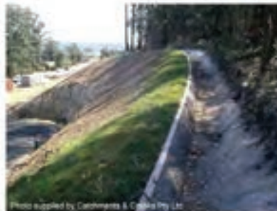
Photo 4 – Permanent catch drain
