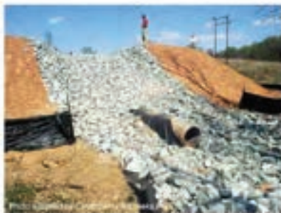
Photo 15 – Emergency spillway located within the fill embankment
