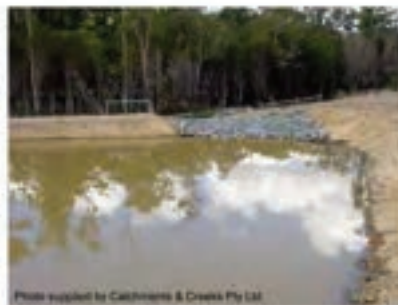
Photo 2 – Type F (wet) sediment basin
