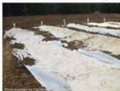
Photo 14 – Sand filter outlet system during installation
