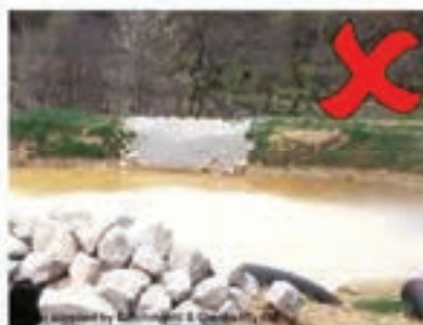
Photo 20 – Spillway crest with inadequate depth or profile
