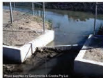
Photo 8 – Litter screen placed on inlet of permanent sediment basin
