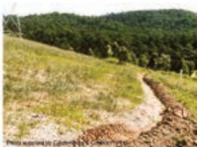
Photo 1 – Unlined catch drain
