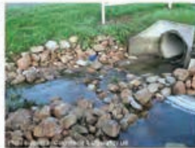
Photo 4 – Rock pad outlet structure
