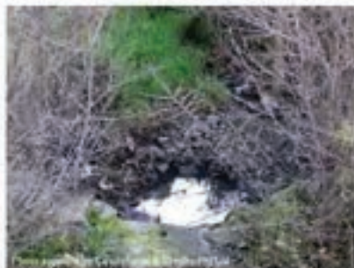
Photo 7 – Rock-lined plunge pool energy dissipater
