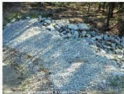
Photo 4 – Rock filter dam with aggregate filter
