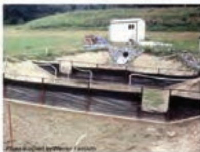
Photo 3 – Inlet chamber can also act as mixing chambers for the addition of flocculants
