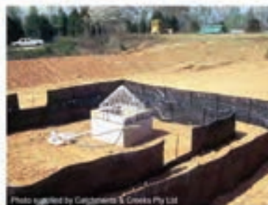
Photo 6 – Outlet chamber surrounding a flexible skimmer outlet device
