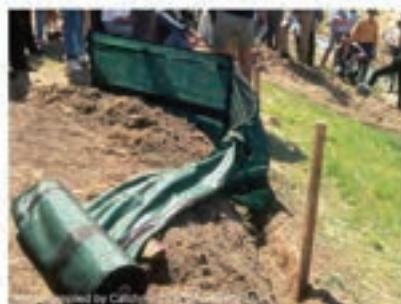
Photo 1 – Installation of a sediment fence
