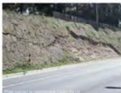
Photo 4 – Slippage of topsoil from steep cut batter
