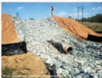
Photo 5 – Spillway chute with well-defined inlet profile
