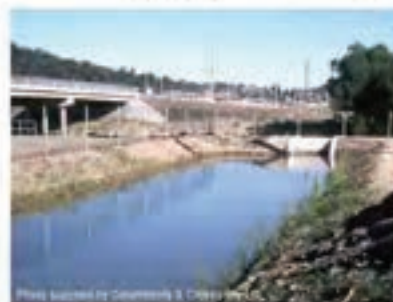
Photo 2 – Example of a 'wet' (Type F/D) sediment basin
