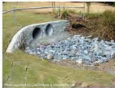
Photo 3 – Rock pad outlet structure
