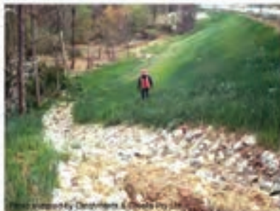
Photo 3 – Rock lined catch drain
