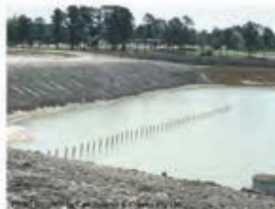
Photo 4 – Internal baffle extending the flow path between the basin inlet (left) and the basin outlet (right)
