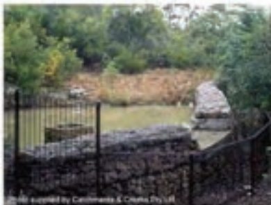
Photo 23 – Permanent sediment basin within residential estate
