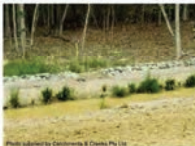
Photo 5 – Sediment trench (with rock filter dam outlet system) located at the base of a fill embankment
