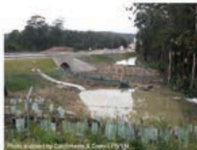
Photo 24 – Sediment basins converted to permanent stormwater treatment ponds on highway project
