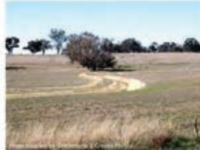
Photo 2 – Large rural catch drain (channel-bank)
