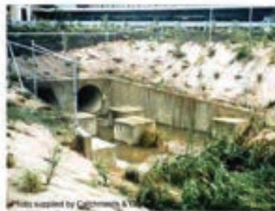
Photo 12 – Impact block energy dissipater
