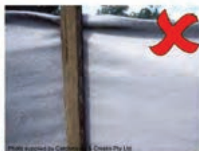
Photo 6 – Filter cloth MUST NOT be used unless used in the construction of a 'Filter Fence' adjacent to a stockpile
