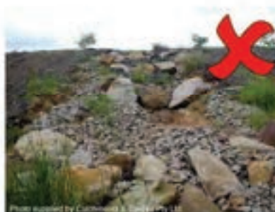
Photo 8 – Erosion caused by inadequate rock size and water bypassing around the poorly located boulders
