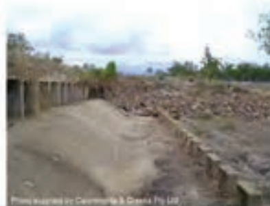
Photo 8 – Note use of impact blocks to stabilise the location of the hydraulic jump
