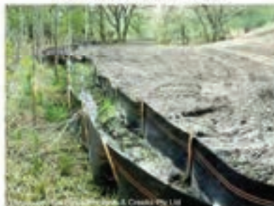
Photo 8 – Double sediment fence
