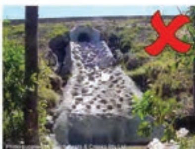
Photo 7 – Severe erosion along edge of chute caused by water spilling out of the chute
