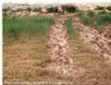
Photo 6 – Rilling down newly vegetated slope cutting through surface roughening
