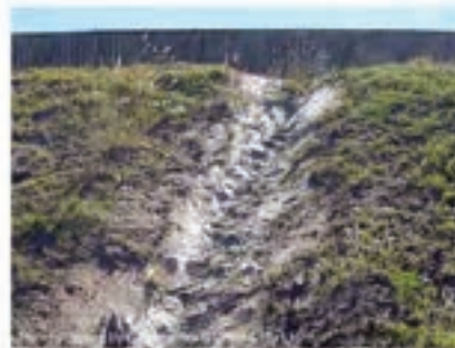
Photo 2 – Temporary batter chute lined with filter cloth
