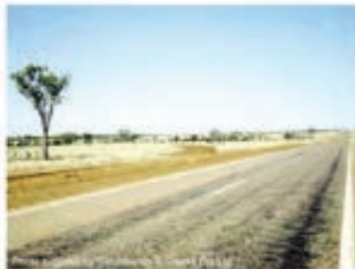
Photo 1 – Diversion drains (centre) collect stormwater from roadside table drains, then releases the water as sheet flow via a level spreader
