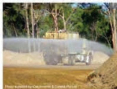
Photo 2 – Dust control using a water truck
