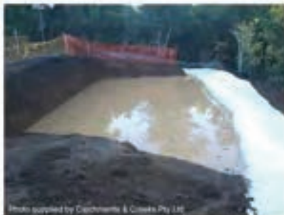
Photo 5 – Recessing the basin into the ground allows the natural ground level to become the spillway
