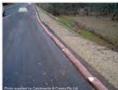
Photo 4 – Sandbag flow diversion berm used to minimise surface flow over a recently seeded embankment
