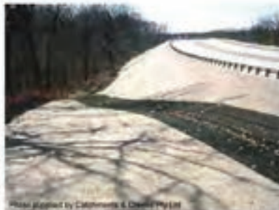
Photo 1 – Application of erosion control blankets and mats
