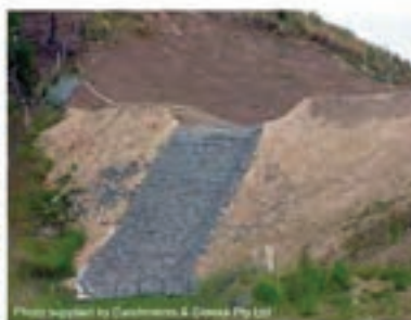
Photo 2 – Rock mattress-lined sediment basin emergency spillway
