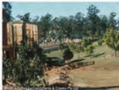
Photo 2 – Flow diversion bank up-slope of a building site
