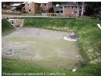
Photo 1 – Type C (dry) sediment basin
