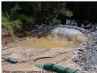
Photo 3 – Rock filter dam with geotextile filter
