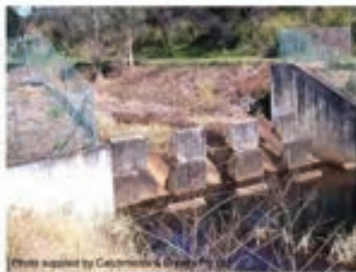
Photo 11 – Baffled spillway
