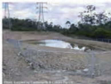
Photo 22 – Temporary fencing of a construction site sediment basin
