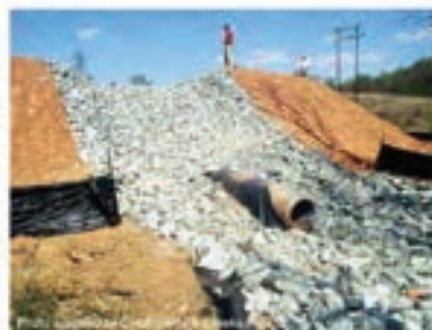
Photo 2 – Rock lined basin spillway and energy dissipater
