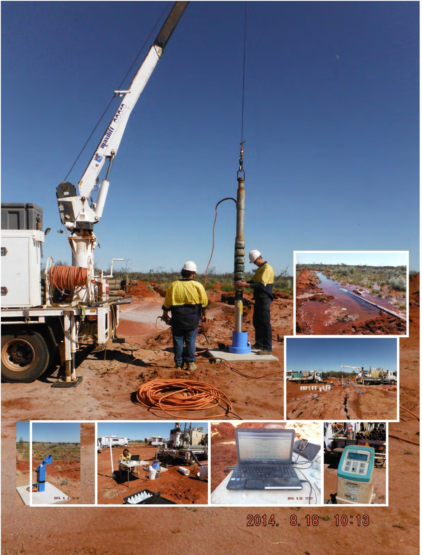
Constant Rate & 4 stage pump test Bore RC # 31 (bore site P1)
