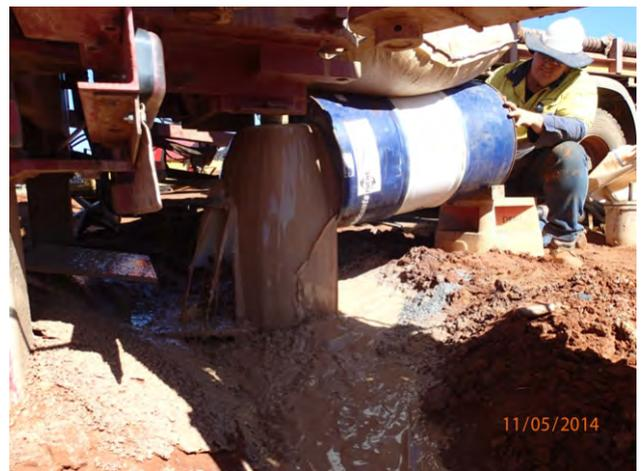
Arafura Reaphook Paleochannel production bores P1, P2 & P6 were drilled as gravel packed or use of a 5 mm aggregate stabiliser with bentonite pellet seal above the stabiliser.
