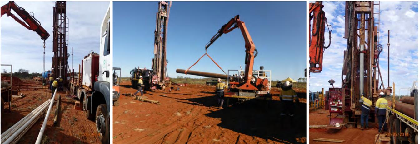
Arafura Reaphook Paleochannel production bores P1, P2 & P6 were drilled as gravel packed or use of stabiliser using Pack R mud circulation and 250 mm ID steel casing and inline stainless steel screens.
