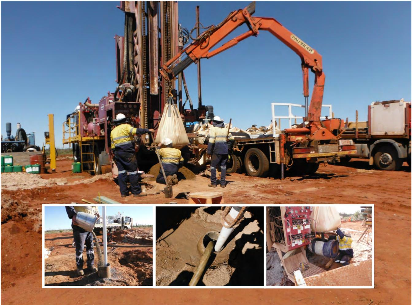
L2 Drillers installing stabiliser from the bulka bags into the annulus between the drilled hole and casing string. A 200 L drum was used to control the flow rate to ensure a complete pack opposite the stainless steel screens.
