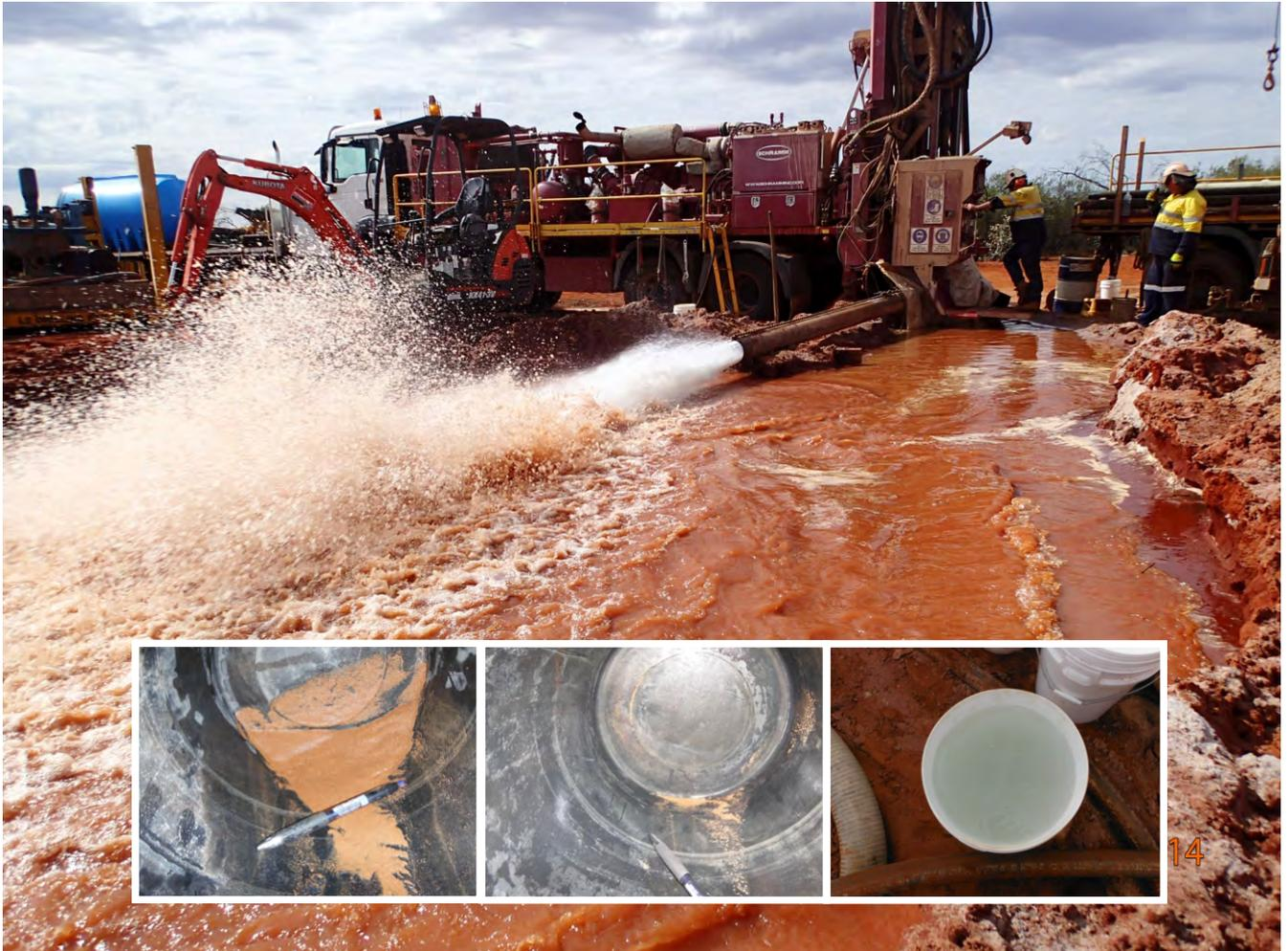
L2 Drillers developing *Arafura* Reaphook Paleochannel production bore P1 to develop removing the fine to medium sand immediately opposite the screens. Required 2 days of development use of a surging tool.
