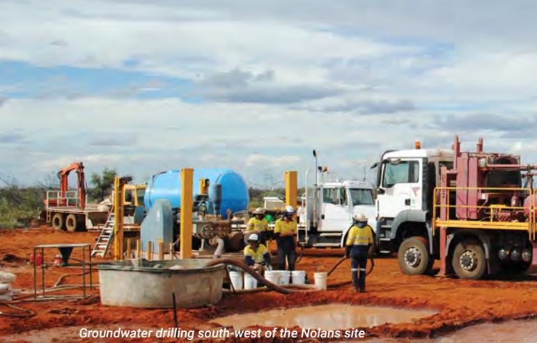
Groundwater drilling south-west of the Nolans site
