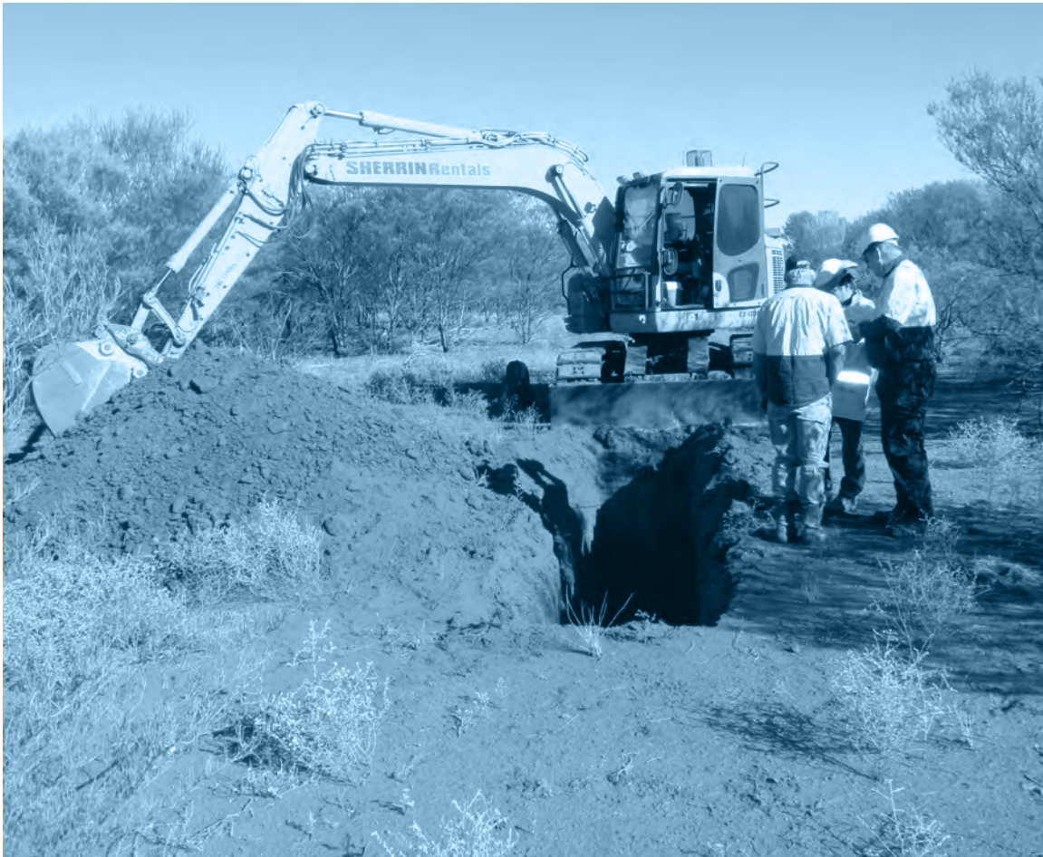
Geotechnical test pit excavation - Nolans process plant site
